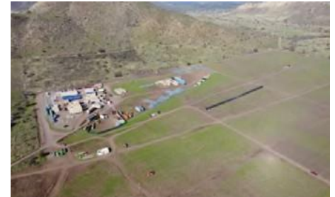
Libélula PV & BESS (350 MW)
