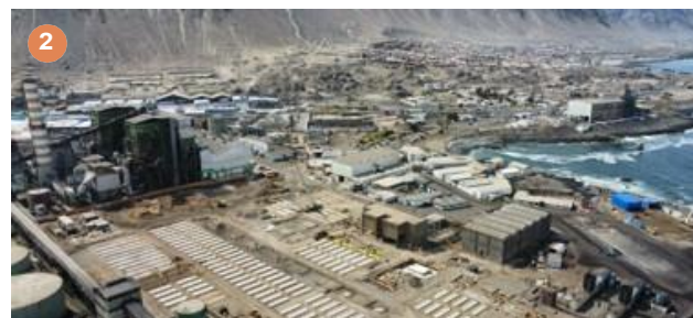
Construction began of Tocopilla BESS, inside our Tocopilla Thermal Power Complex. It will have a storage capacity of 600 MW/h and is our first stand-alone storage system that operates independently and is connected to the transmission system to inject energy.
