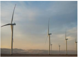
163 MW Calama wind farm
