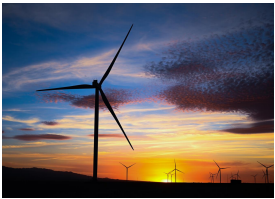
344MW Kallpa wind farm
