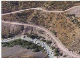
1 MW Cosapilla Hydro
