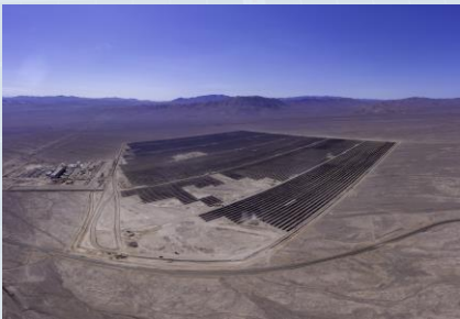
76MW / 418 MWh BESS Tamaya (storage)
