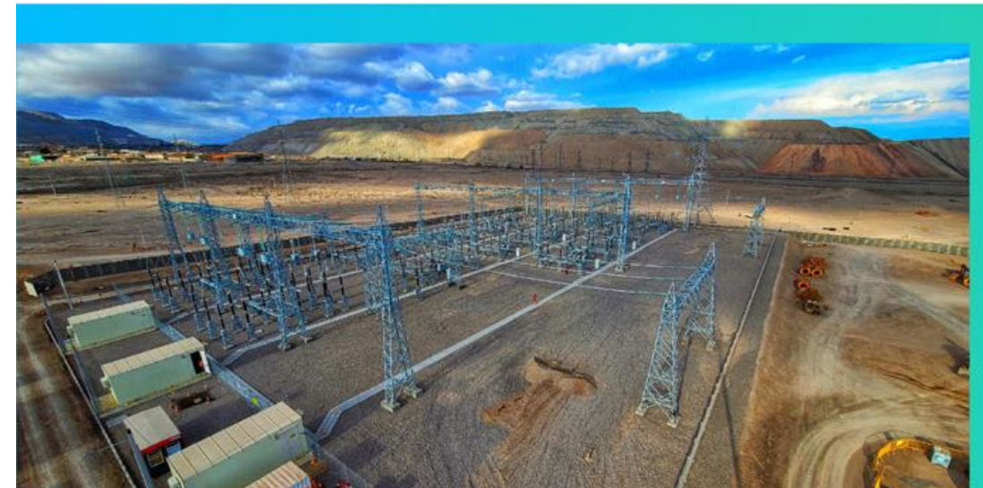
Nueva Chuquicamata (National) Substation +2 x 220 kV transmission line COD: SS: Completed / TL: energization upon Calama SS commissioning – Nov-21
