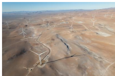
57MW BESS Kallpa US$69 million CAPEX COD(e): 2H2026
