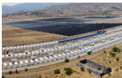
350MW PV+BESS Libélula US$320 million CAPEX COD(e): 2H 2026
